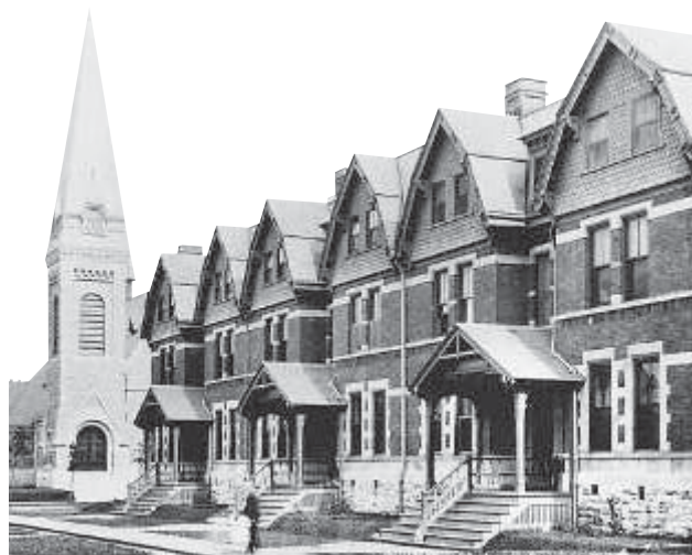
▲ The town of Pullman was carefully laid out and strictly controlled.
